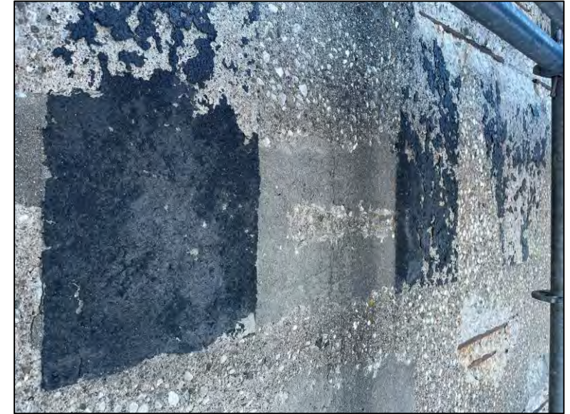
The original tar paper installation.
