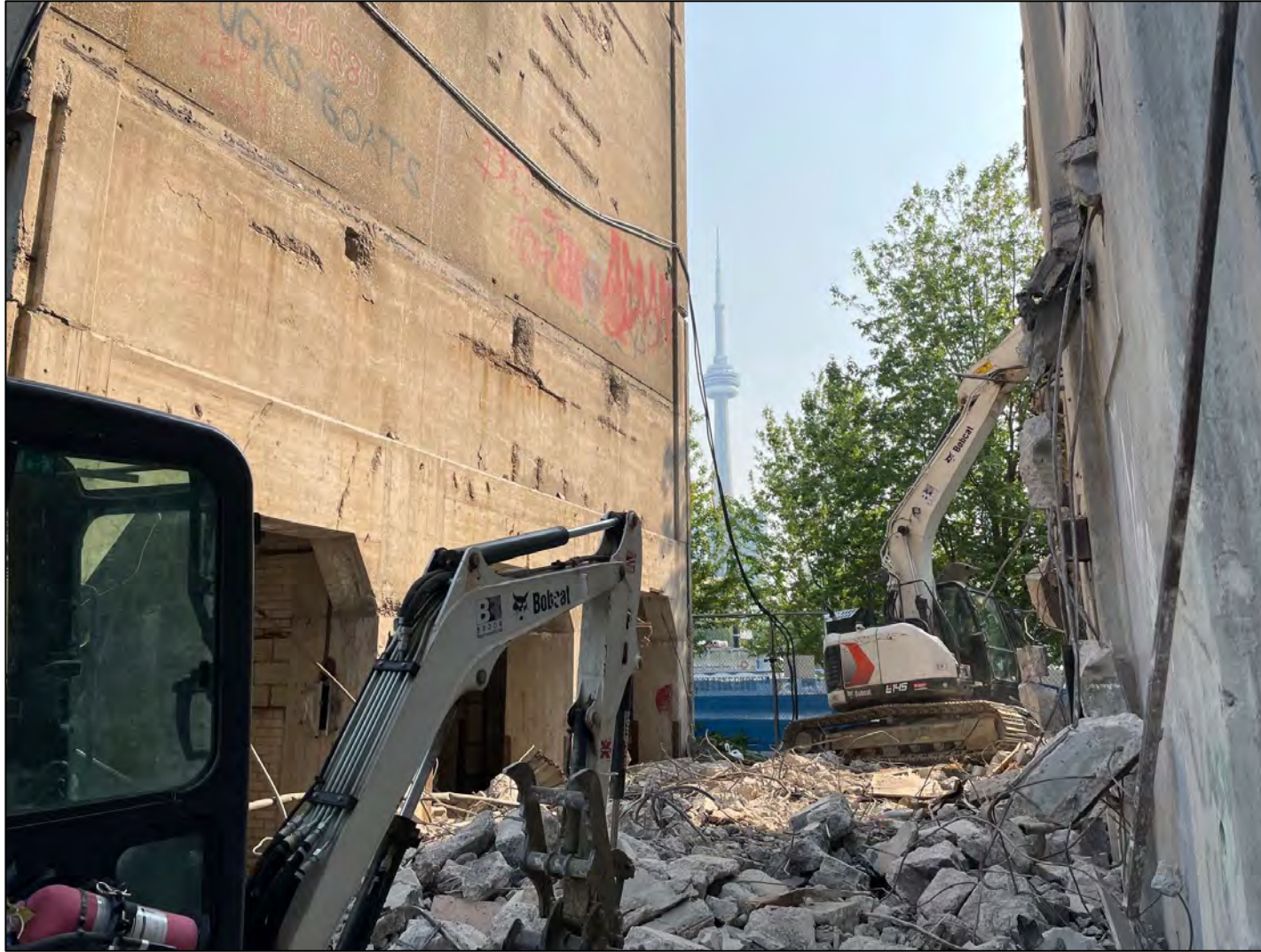
Demolition to create roughed in silo 'portal'.
