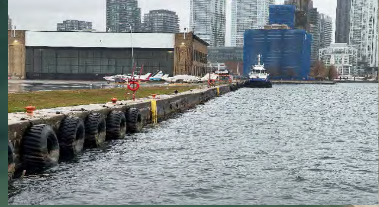
Island East Dockwall Rehabilitation
